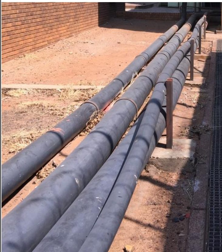
Figure 7: Steel Pipe Supports
