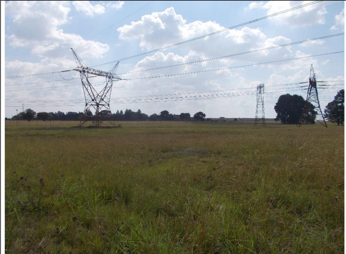
Figure 14: Representative photograph of the artificial wetland traversed by alternative 2.
